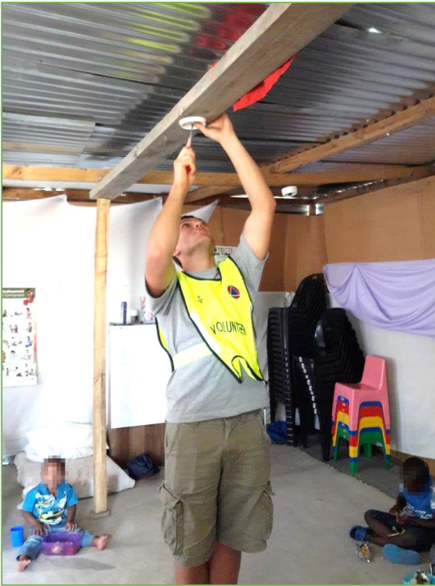
Figure 10 SU student assists installing a smoke alarm in an informal dwelling as part of IDDR 2017 outreach
